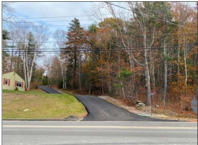
Pine Woods Road After - Newly paved road surface with armored ditches and turnouts
