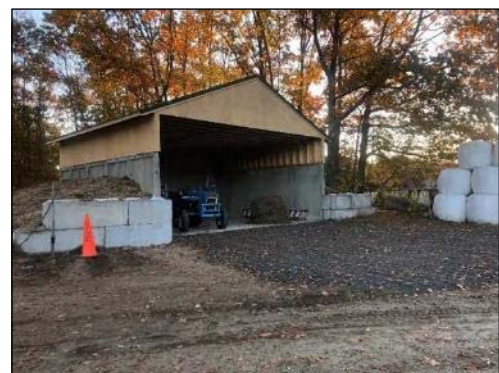
Manure storage shed and heavy use area constructed at Down Home Farm. NRCS provided input on project design.
