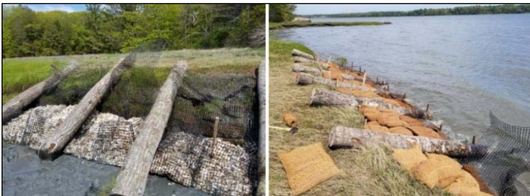
Maquoit Bay Living Shoreline Demonstration Project – To stabilize the eroding high marsh edge, Tensar GeoReef baskets were tucked under logs and filled with oyster shell. Coir bags were staked into place above the baskets. Photo credit: Maine Geological Survey
